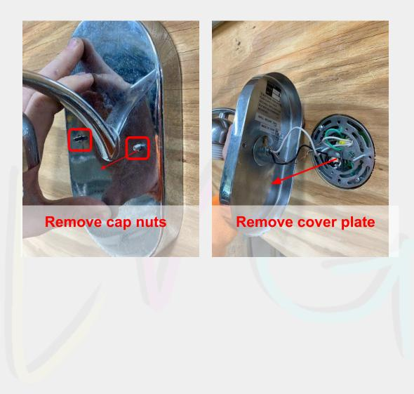
Unscrew any screws/bolts securing the lighting bracket to the junction box. Depending on the type of screws you may be able to just loosen them.
